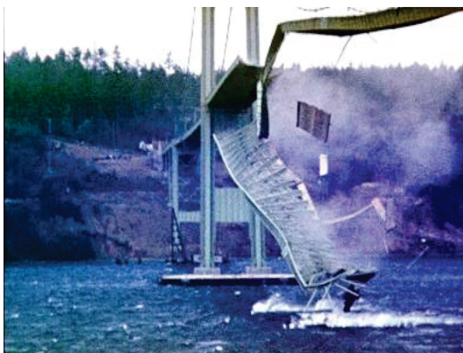
Fig.3-16; Vibrations breaking the bridge
